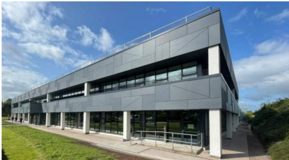
Melbourn Building, MTU Cork Bishopstown campus, after retrofit
